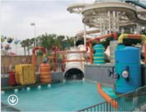
Water Park Ride Landing Pool Major new water ride ends in exploding water pool
